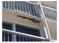
This component allocates funds to perform concrete and spall repairs, and is scheduled to coincide with the exterior painting project. The actual amount of spall repair cannot be determined based on a visual observation, and the extent of the spall and concrete repairs continually change based on exposure to natural elements.
