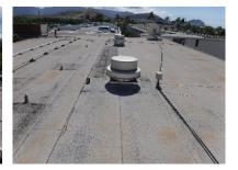
There is approximately 64,000 square feet of roofing over the buildings, conference room, fitness room/restrooms, entry, guard shack, BBQ area, etc. This component allocates funds for a fluid-applied roof coating system for the main tower, elevators, and staircases.
