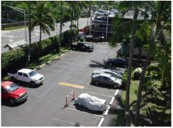
There is approximately 22,000 square feet of uncovered asphalt. The useful life of an asphalt seal coat is typically longer when protected from natural elements and when proper drainage is maintained.
