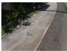
According to Makaha Surfside representatives, all buildings are post tension, and brace supports were added to Building B. This component allocates funds to perform concrete and spall repairs throughout the property. The actual amount of spall repair cannot be determined based on a visual observation and the extent of the spall and concrete repairs continually change based on exposure to natural elements.
