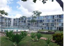
This component allocates funds for exterior painting of Building C. It is scheduled to coincide with the exterior concrete spalling/repair project. This component also allocates funds to scrape portions of the existing paint that may have begun peeling, or may have become thick enough to cause delamination from the concrete surface in some areas.
