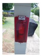
There are approximately 58 extinguishers throughout the property. According to Makaha Surfside inspection tags, the most recent test was completed in August 2018. This component assumes the fire extinguishers are replaced as needed and covered as an operational expense.
