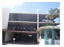
There is approximately 3,500 linear feet of steel garage cabling. This component allocates a repair fund to repair and replace the the garage cables as needed. It is unknown if these are post tension cables.
