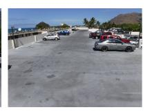
There is approximately 39,400 square feet of coating on the parking deck. This component allocates funds for a new coating system for the parking garage deck. Repairs will be required
