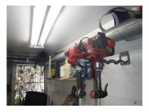
According to the Makaha Surfside inspection tag, the most recent test was completed in May 2021. The required frequency is unknown but is believed to be every five years. There are 10 functional standpipes. Per conversations with Makaha Surfside representatives, 2 of the stand
