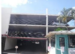
This component allocates funds to perform concrete and spall repairs, and is scheduled to coincide with the exterior painting project. The actual amount of spall repair cannot be determined based on a visual observation, and the extent of the spall and concrete repairs continually change based on exposure to natural elements.
