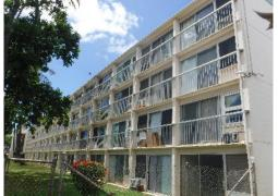
There is approximately 4,005 linear feet of railings in the corridor and 5,350 along the lanais. This component allocates funds for corridor and lanai railing replacement. This component allocates funds in conjunction with the building painting and spalling projects.
