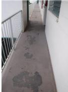
There is approximately 42,000 square feet of coated walkways along the corridors. This component allocates funds to coat the corridors as needed. This component assumes the concrete spall repairs will be repaired during the building painting project.
